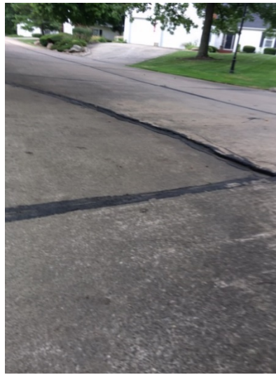
Another example of a sunken concrete slab.
