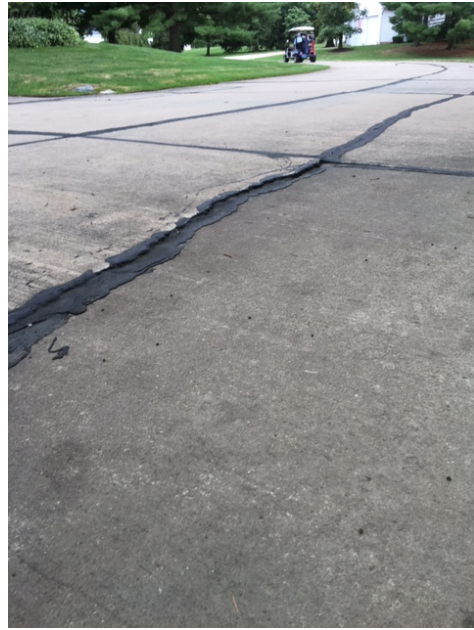
An example of a sunken concrete slab needing replacement due to uneven heights.
